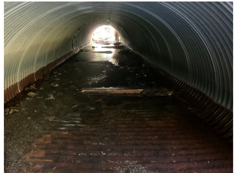
Looking Downstream Through CMP
